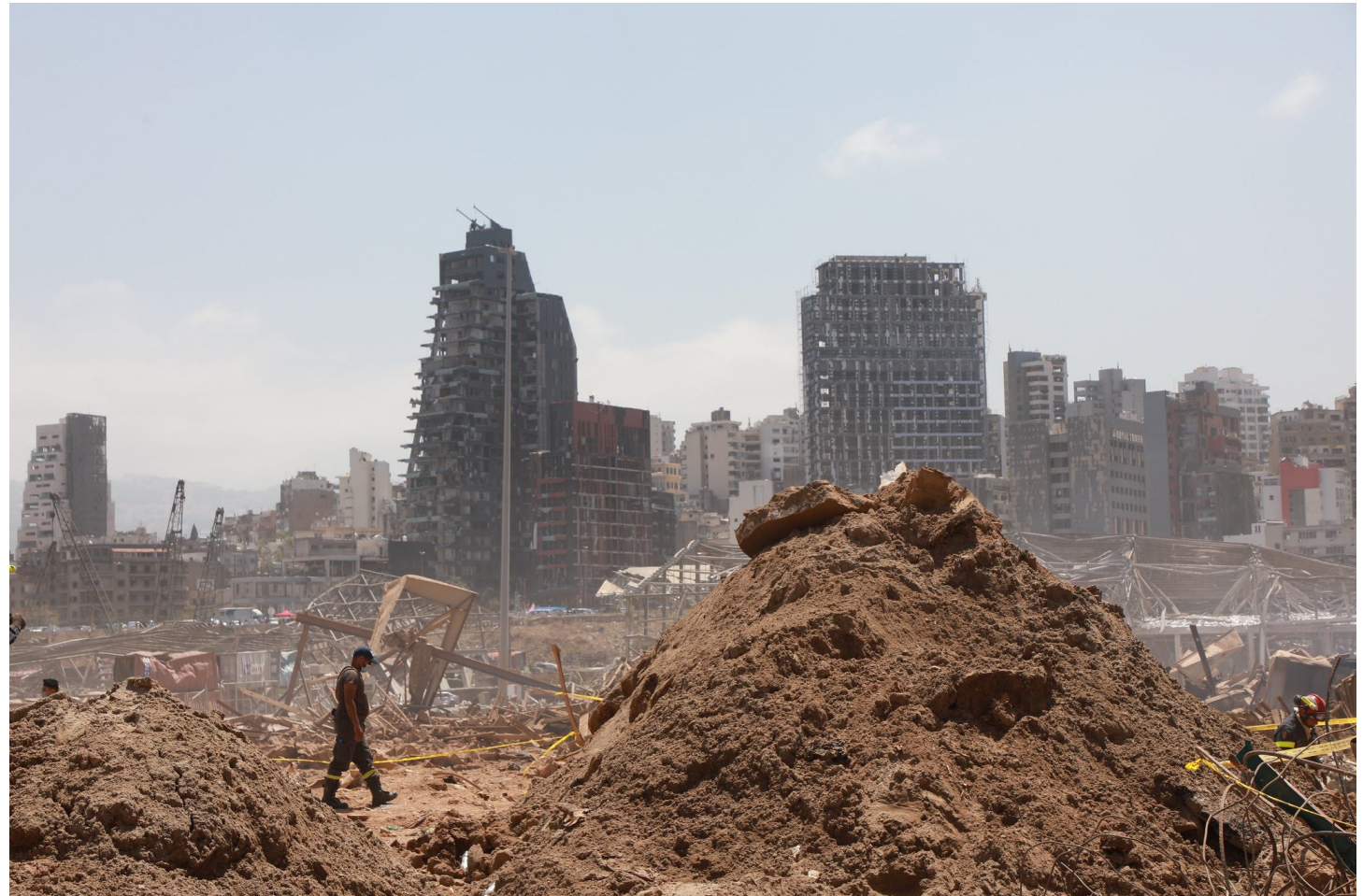
Seaport of Beirut on August 8, 2020; Image credit: European Union (photographer: Bernard Khalil)
